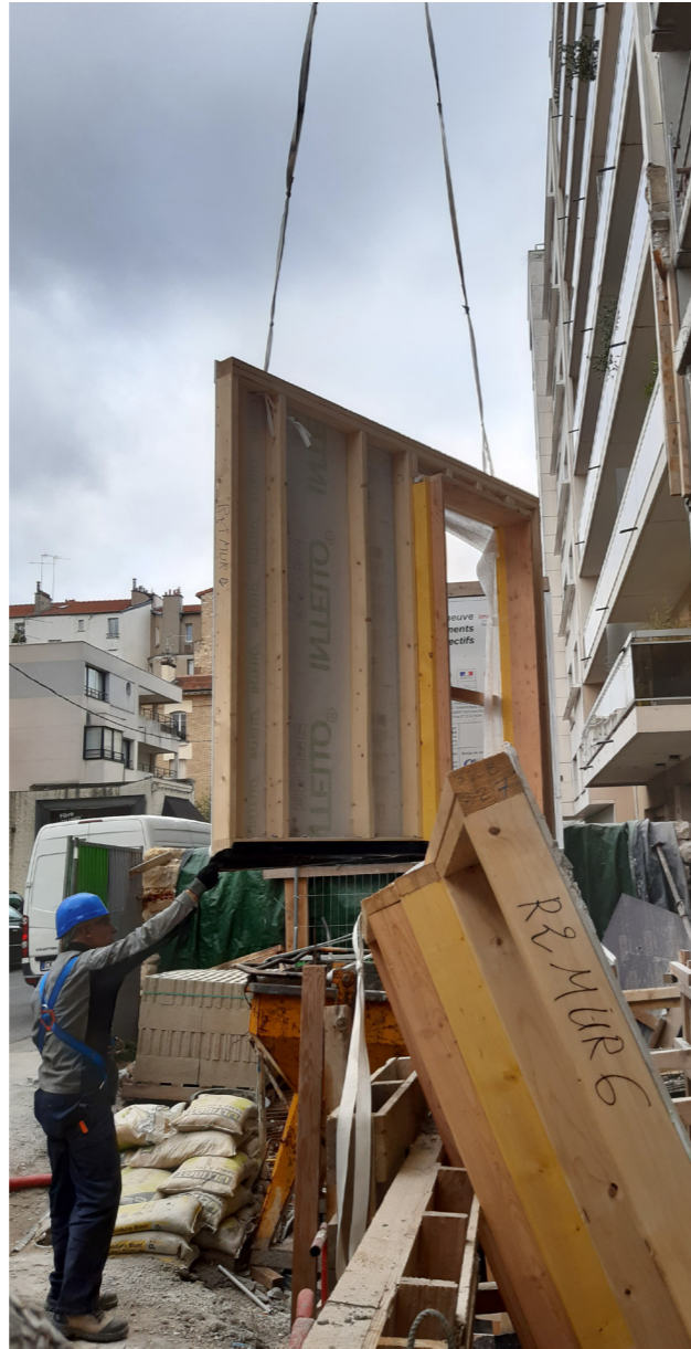
Fig. 11: Facade units © North by Northwest Architectes
