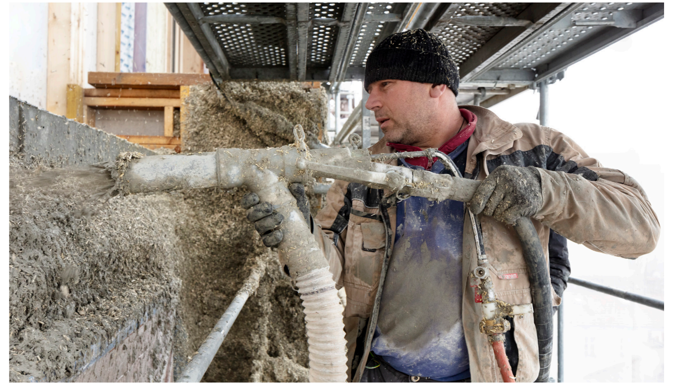
Fig. 9: Pouring Hempcrete at construction © CecileSeptet
