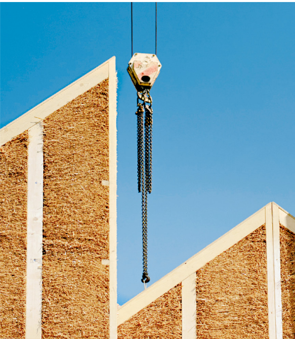
Maison en Finlande, EcoCocon, Natural Building Company.
